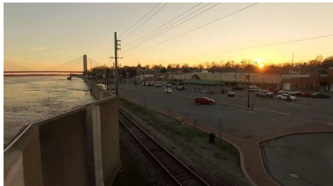
Cape Girardeau Floodwall
